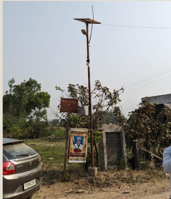
Solar panels and CCTV installed
