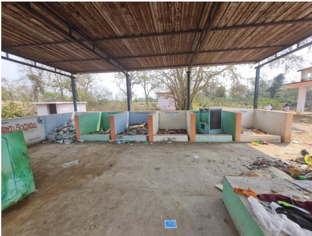
Photo: Pictures of waste segregation shed in the village
