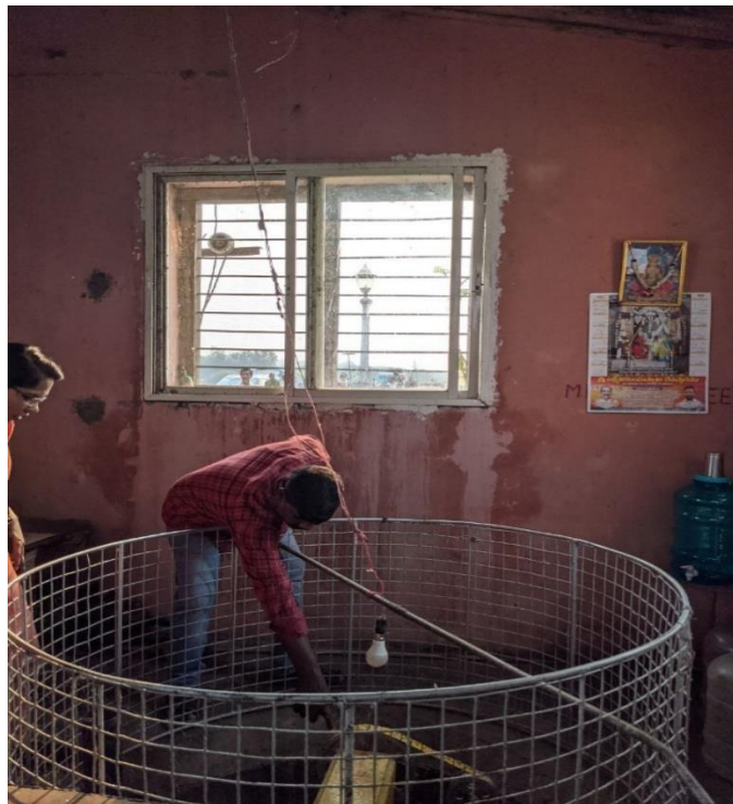
Photo: Water lifting infrastructure at the Kadam Project site
