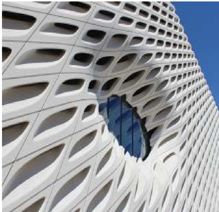
Fig: Glass Fiber Reinforced Concrete (GFRF)
