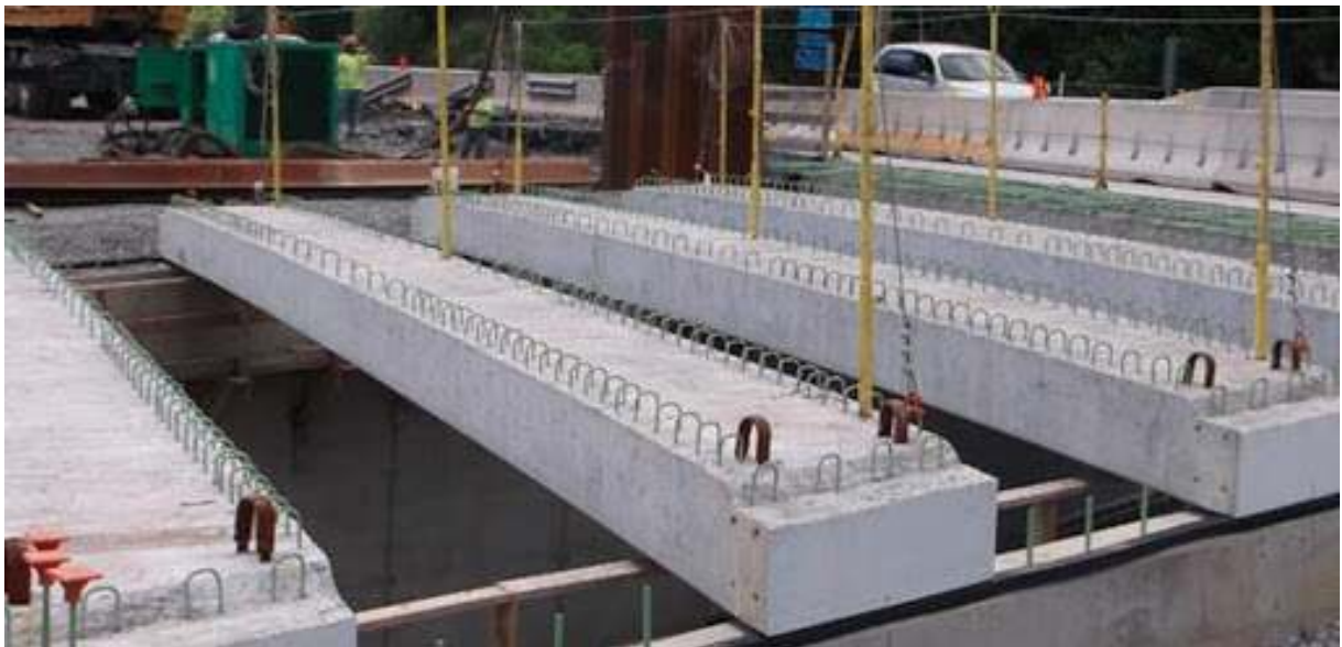
Fig: Prestressed beams
