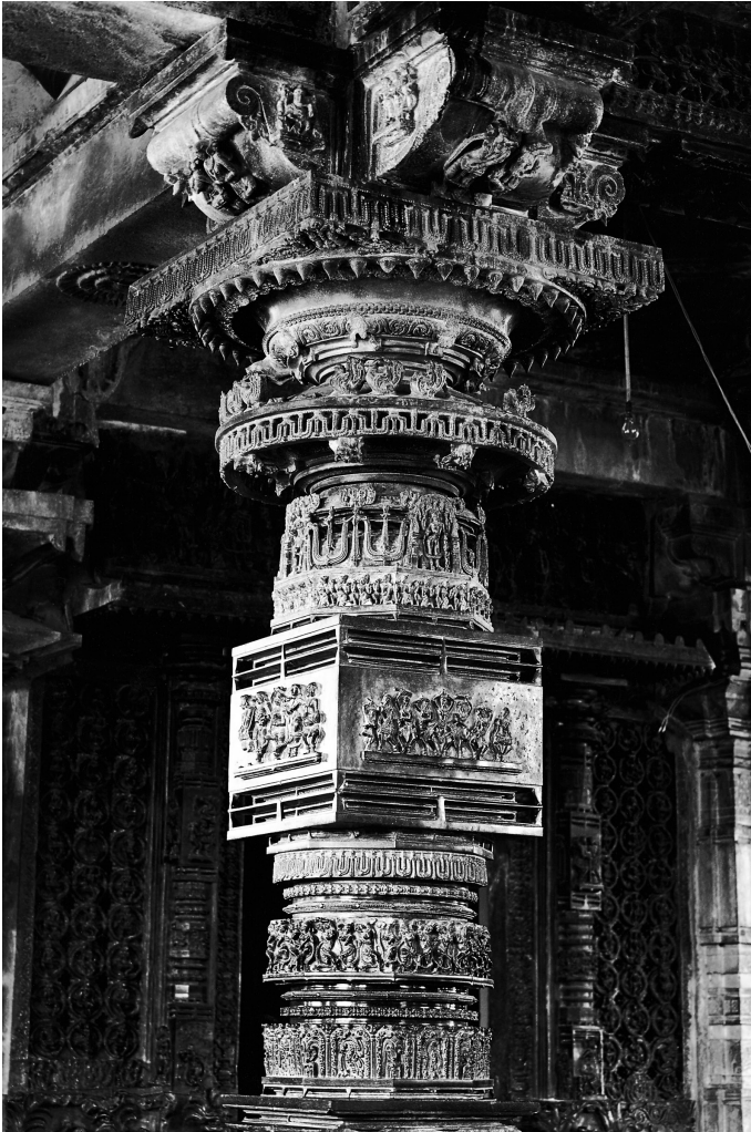
Kakatiya Pillar, Ramappa Temple, Warangal – The finely sculpted and highly decorated pillar in black granitic stone is one of the four pillars that support the main mandapa of the temple. 1213 CE, Recherla Rudrudu, Kakatiya period
