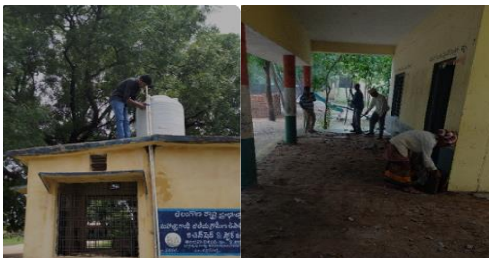
On-going infrastructure repair works
