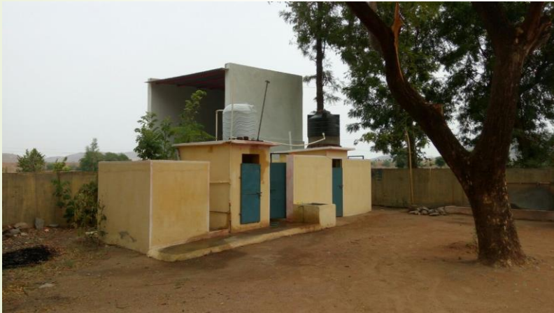
School Toilet with water facility
