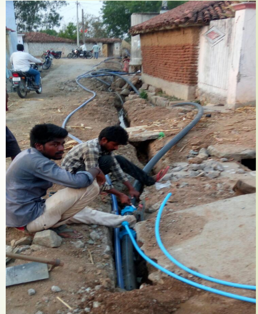
Work in Progress for laying Water cables
