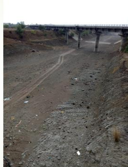
SRSP FLOOD CANAL
