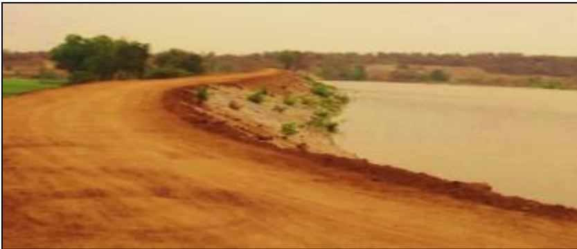
Restored Tank Bund
