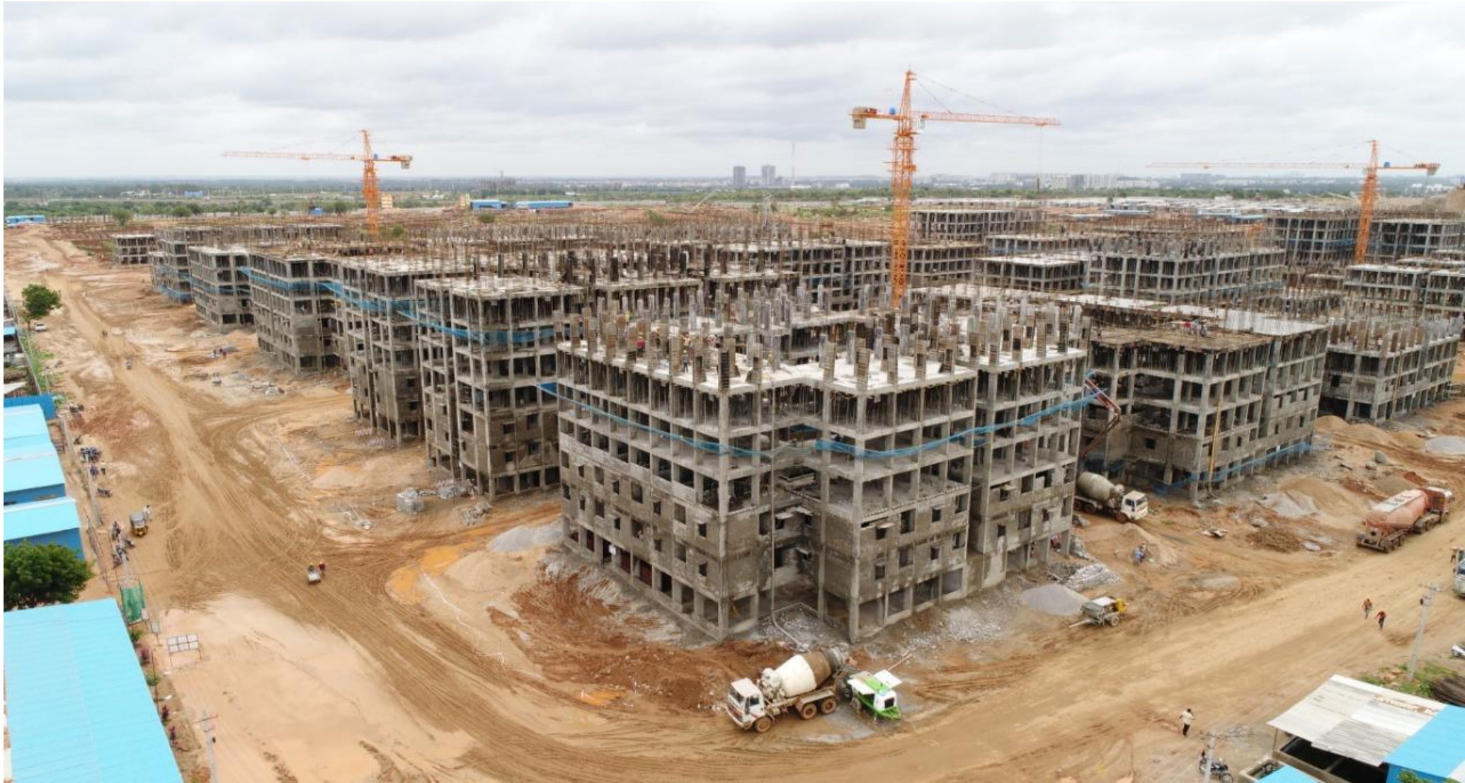
15,660 houses in-progress - Kollur, GHMC
