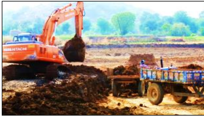
Desilting of the Tank
