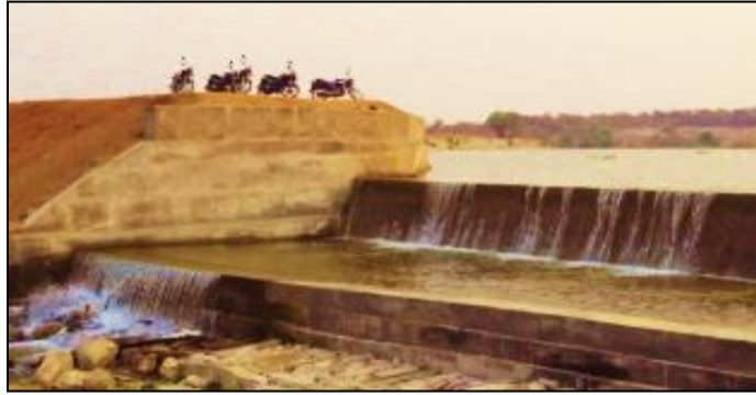
Restored Surplus Weir
