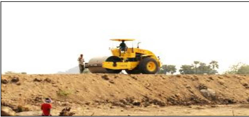
Strengthening of Bunds
