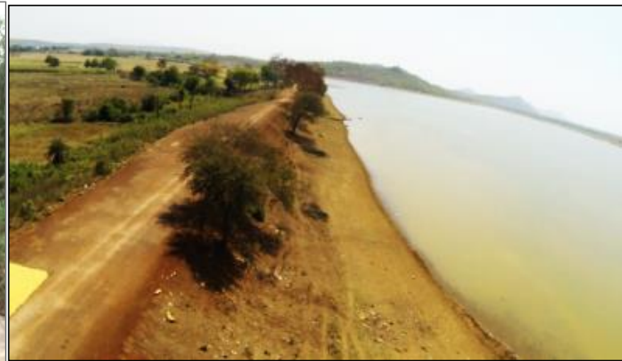
Improved Water Level in Restored Tank
