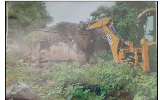
Demolition of Abandoned Houses
