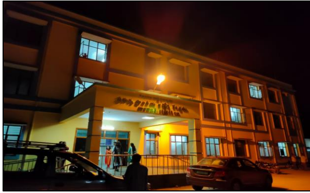
Well Structured Building
