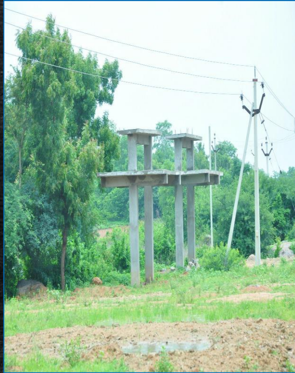
Crematorium (Under construction)
