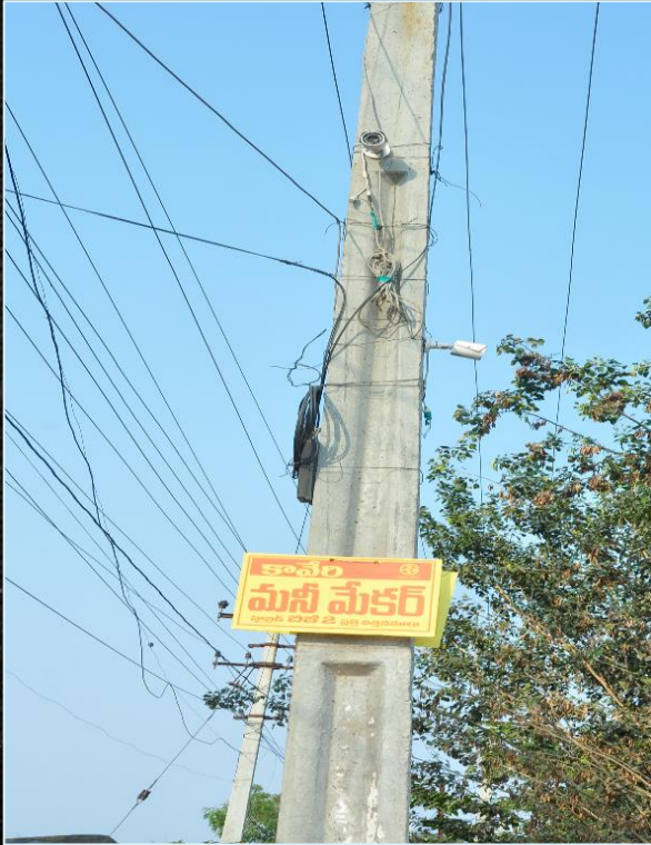
28 CCTV Cameras with Centralized Monitoring
