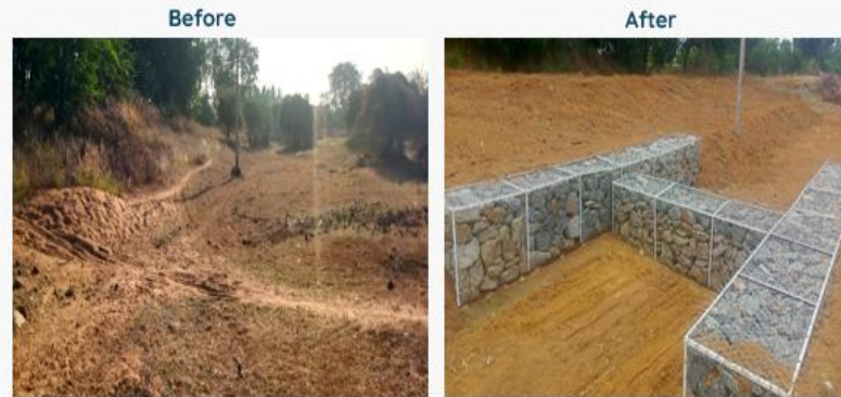
Gabion structure-1 at supply channel in Pappankulam village
