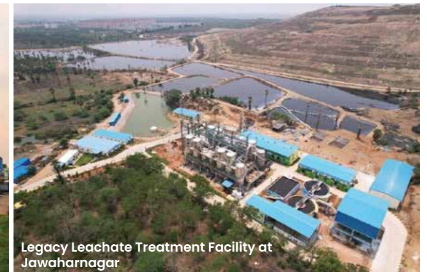
Legacy Leachate Treatment Facility at Jawaharnagar
