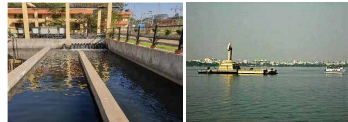
20 MLD STP with Tertiary Treatment adjoining HussainSagar Lake, Hyderabad
